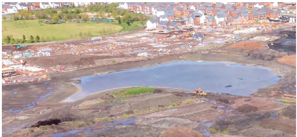
AERIAL IMAGE OF THE CENTRAL LAKE BEING FORMED
